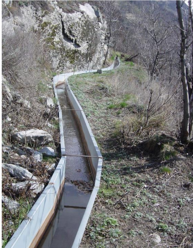
Photo: Aluminiumkanal / chenal en aluminium Laldneri – Eggerberg
