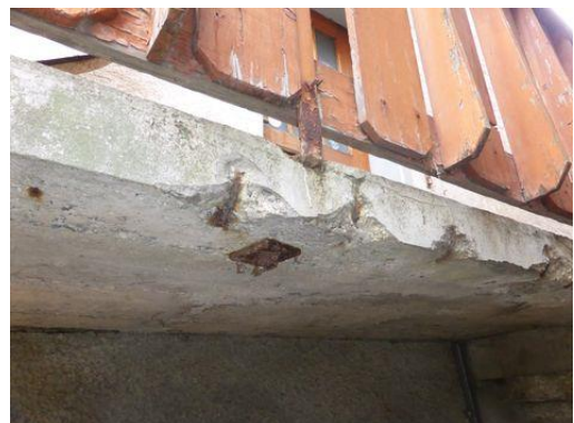
Carbonatation dalle
