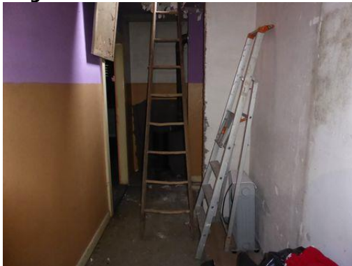
Couloir de distribution
